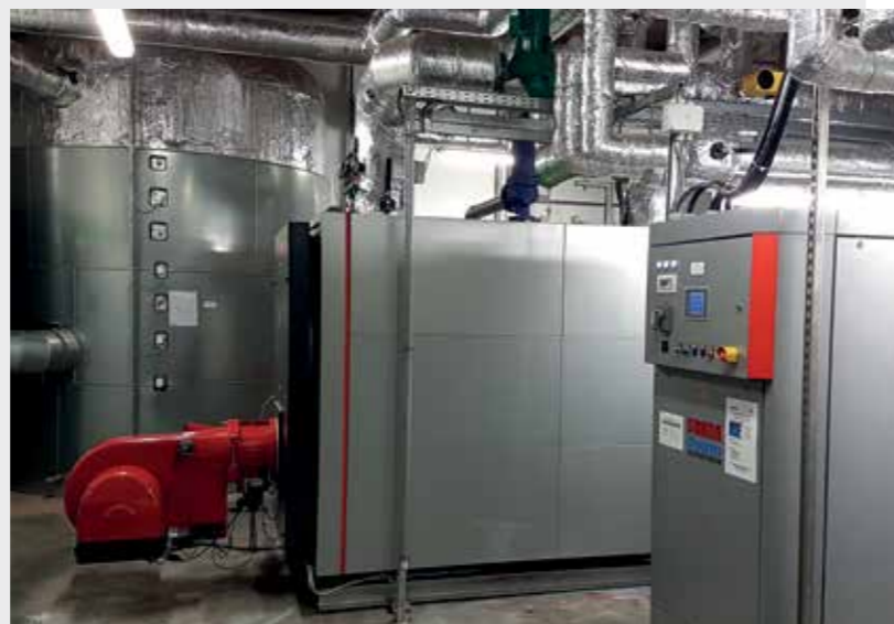
Two cogeneration plants cover 50 % of the factory's need for power. The inevitable heat produced is used for heating water and buildings, and for drying leather.
